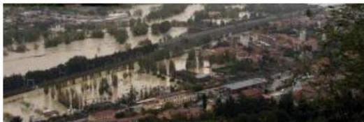
Paglia river Flood damage 2012
