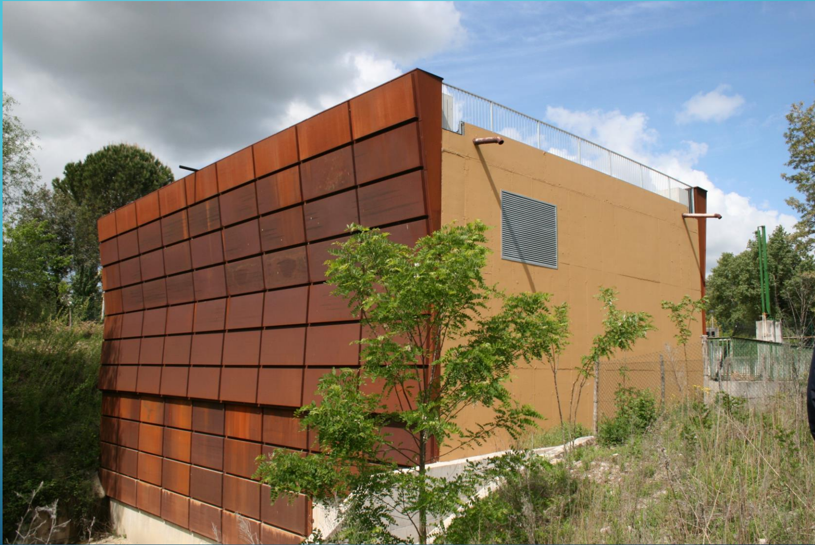
Power station buildings
