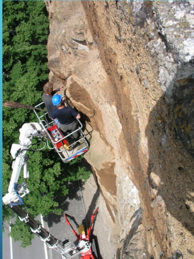
Tuffaceous wall maintenance
