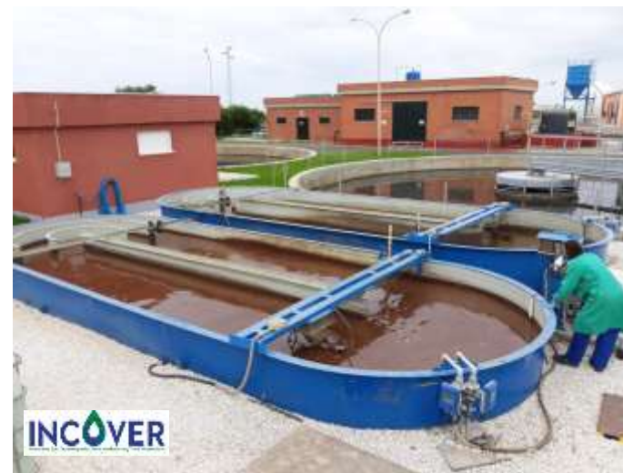
PHOTOTROPIC PURPLE BACTERIA CULTIVATED TO RECOVER PHA
