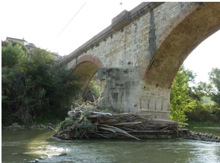
Pontecuti Bridge – Tiber River
