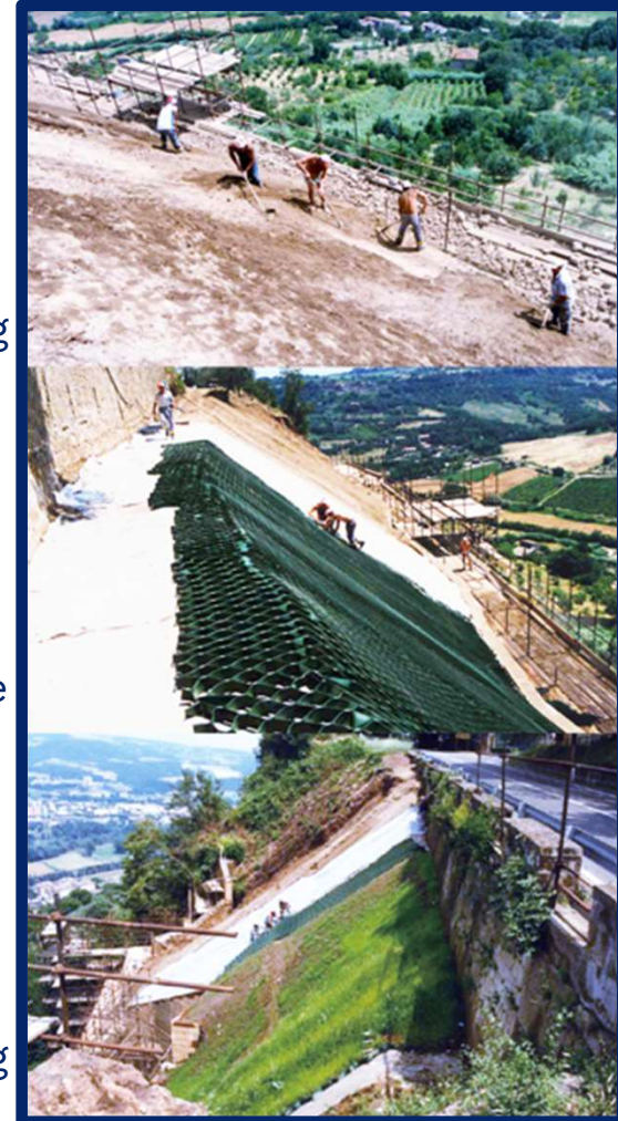
Placement of geotextile
