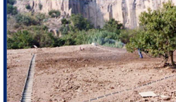
Prefabricated channels
